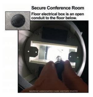
As shown in the photo, acoustical leakage is often caused by small construction oversights, which later become big information security vulnerabilities.
